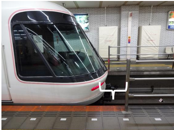
Photo 1. The clearance between the falling prevention fence and the front carriage of the train (Osaka-Abenobashi, Kintetsu Railway)
